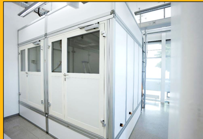
Class 1 dry cleanroom (ISO 14644-1) with relative humidity < 1%
